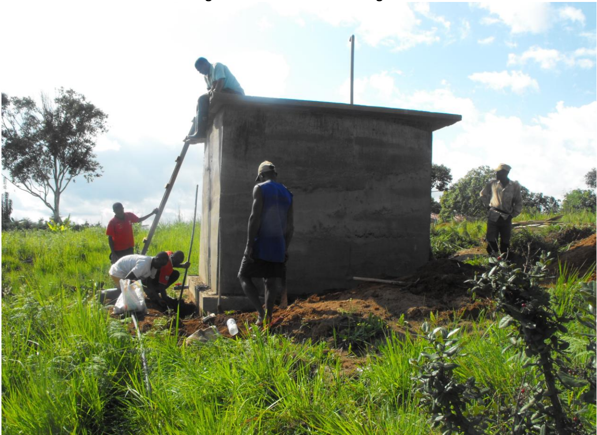
Betonwassertank in Batack-Bavouantou.
